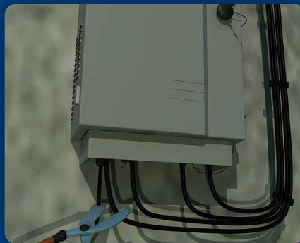
RF Cables Cut Off Deliberately
